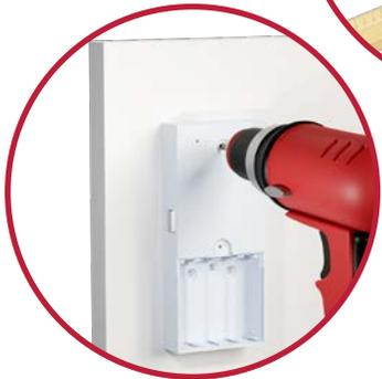
Carefully drill 4 pilot holes for the mounting screws.
