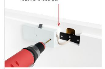
Drill pilot holes for the mounting screws.
