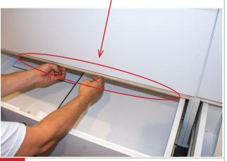
Slide the drawer to a nearly closed position and lightly mark the location where the lock bolt meets the underside of the cabinet. (This is for positioning the lock latch assembly.)
